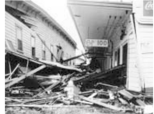
Damage to buildings in Hilo, Hawaii, from the 1946 tsunami. Credit: Pacific Tsunami Museum
