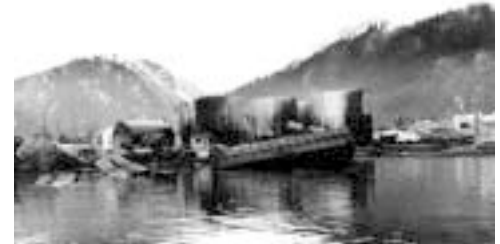
Damage to port facilities in Seward, Alaska, from the 1964 tsunami. Locating industrial facilities outside of inundation zones is the most effective mitigation technique. Credit: U.S. Army Corps of Engineers
