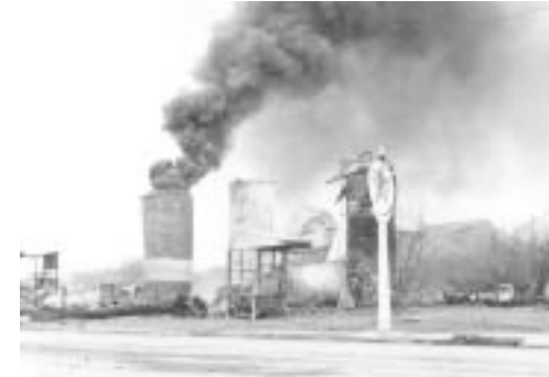
Petroleum tank on fire due to damage from the 1964 tsunami on Highway 101 near Crescent City, California. Credit: Del Norte Historical Society
