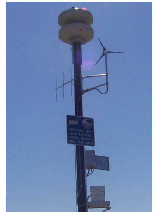
Prototype installed in Ocean Shores July 2, 2003
