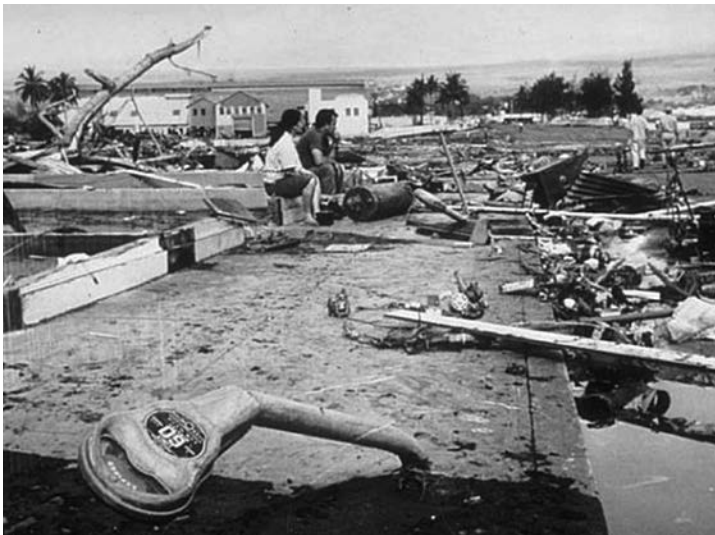
Hilo, Hawai'i. The tsunami that struck Hilo on May 23, 1960 was caused by a magnitude 9.5 earthquake off of Chile the day before. Water and debris carried enough force to crush wooden buildings and twist parking meters by the time it hit Hilo 15 hours later. Photo courtesy of NOAA/NGDC and the Pacific Tsunami Museum.
