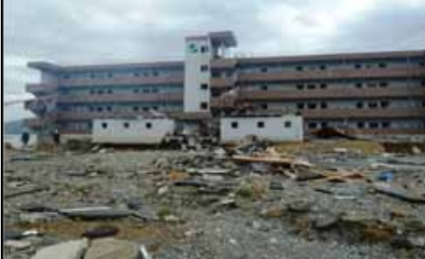
Concrete building survived tsunami, but roof evacuation area inundated by 0.7m water
